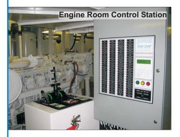
The IMACS workstations and Omni Chief units, featuring layered redundancy with an redundant high-speed network connectivity, function independently without a centralized file server. The IMACS can summarize and network all the data that is collected from electronic engine packages, fire alarm panels, power management systems, motor controls, environmental controls and other electronic control systems throughout the vessel.
